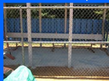
Brick dugout floors – Ailey Young Park
