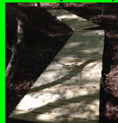
Swamp trail walkway - Camp Agape
