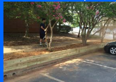
Retaining wall – Our Lady of Lourdes
