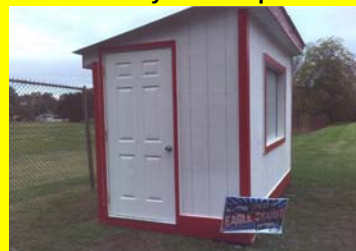
Renovate concession stand - Masonic Home for Children
