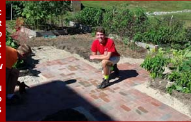
Cross-shaped walkway – Christ the King Lutheran
