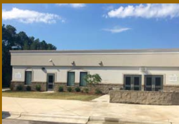
Removed wall – Christ Community Church
