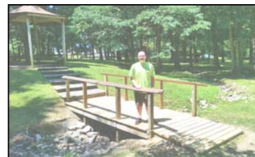
Bridge restoration – Harper Park (Knightdale)
