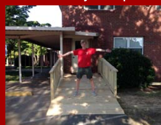
Wheelchair ramp – Salem Baptist Church
