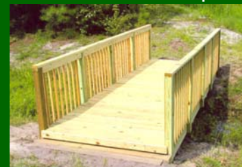
Bridge – Cape Fear High School
