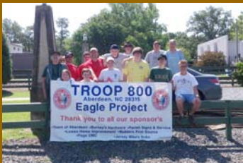
Fence repair, painting – Town of Aberdeen
