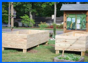
Raised planters – Highland United Methodist
