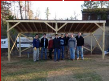
3 shelters – St. Michael the Archangel
