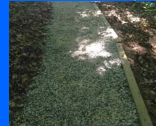
80-foot trail – Benson Memorial Methodist Church
