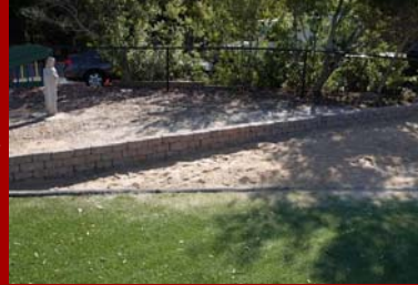
18" retaining wall – St. Michael Early Childhood Center
