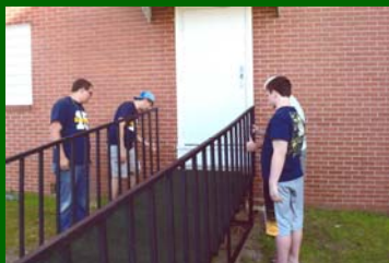
Refurbish wheelchair ramp – Concord Baptist Church
