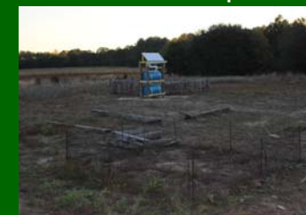
Rainwater collection system – Crossroads Church
