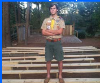
Amphitheater repair – A. B. Combs Elementary
