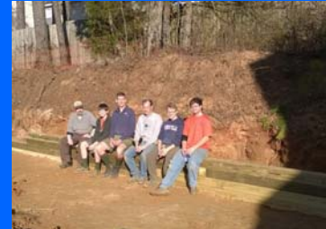
Retaining wall, drainage – Habitat for Humanity
