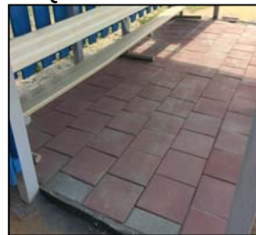
Brick dugout pavers – Tyler Run Park (Wake Forest)
