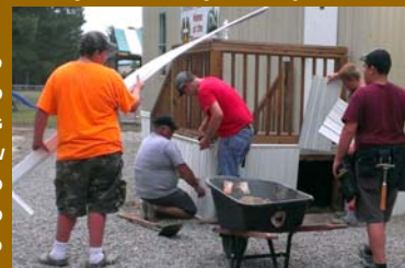
Stairs – New Covenant Fellowship Church
