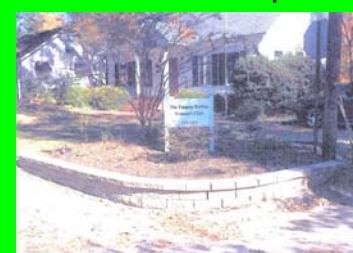
Retaining wall - Fuquay Varina Women's Club
