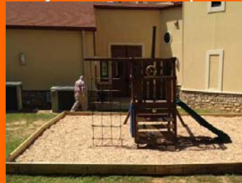
Playground staining – St. Barbara Church
