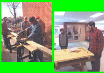
Picnic tables repair – Optimist Farm
