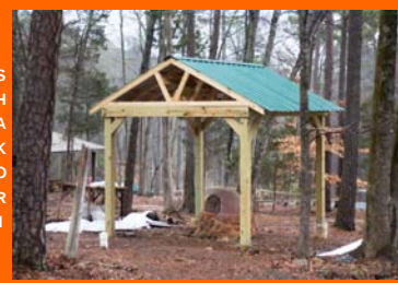
Bread oven shelter – Emerson Waldorf School
