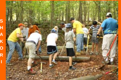
Erosion controls – Eno River State Park
