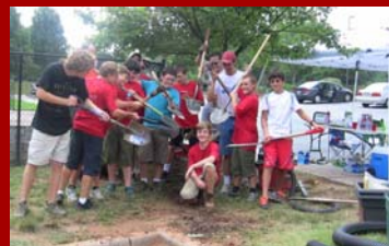
Drain pipe, basin – Genesis Methodist Church
