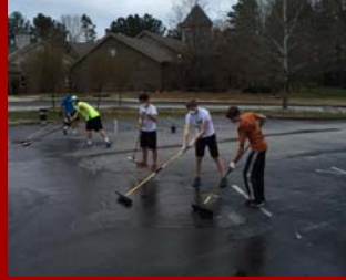
Resurfacing parking lot – St. Andrew's
